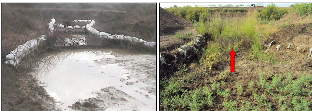
Technology (Brushwood inlet spillway) developed under NAE programme for the protection of inlet of farm pond
